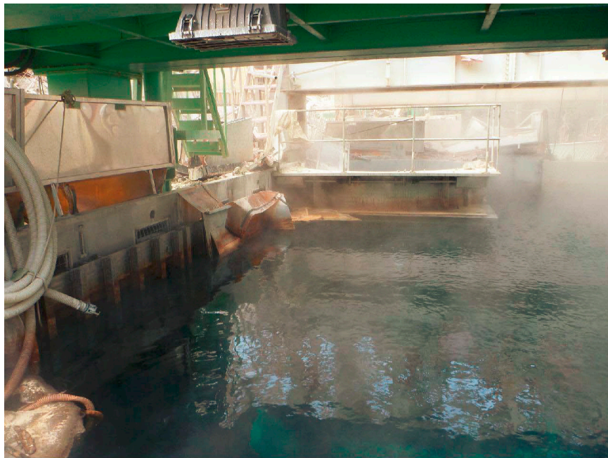
FIGURE 2B.2 Water evaporating from the surface of the Unit 4 spent fuel pool. SOURCE: TEPCO image released June 29, 2011.
