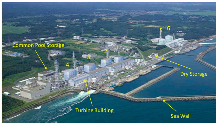
FIGURE 2.1 Oblique aerial photo of the Fukushima Daiichi Nuclear Power Station prior to the March 11, 2011, earthquake and tsunami. Note: Spent fuel was being stored in the Unit 1-6 reactor buildings, the common pool, and in a dry cask storage facility. SOURCE: Photo courtesy of TEPCO.
