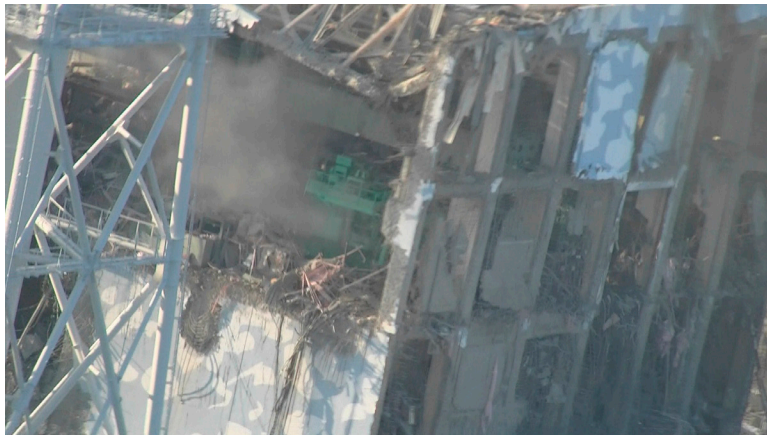
FIGURE S2.1 Photograph of Unit 4 obtained during the March 16, 2011, helicopter overflight of the Fukushima Daiichi site. The photo shows the refueling deck region in the vicinity of the spent fuel pool. The green equipment visible in the center of the image is the fuel handling machine. SOURCE: http://photo.tepco.co.jp/en/date/2011/201103-e/110317-01e.html .
